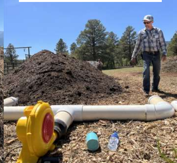
Aerated Static Pile Construction
