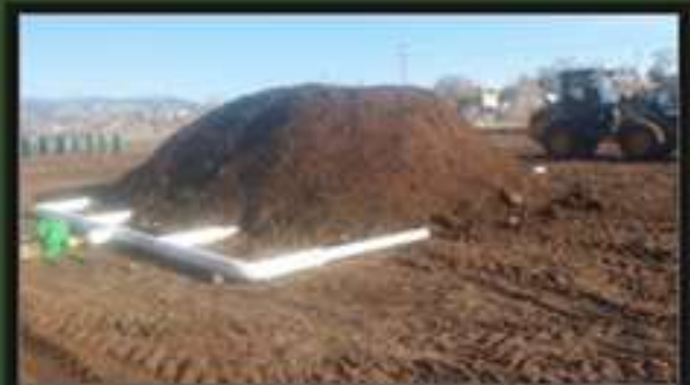
One of our Aerated Static Piles.
